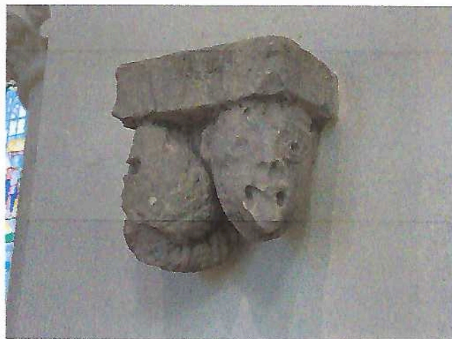
Fig 8b relocated corbels from roof
